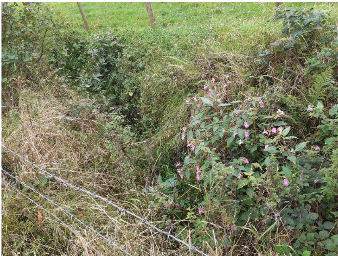
Photograph 3: Western drainage ditch, lined by hedgerow and frequent Himalayan balsam. (TN 3)
